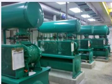
Wells Sanitary Blower Motors for Aeration
