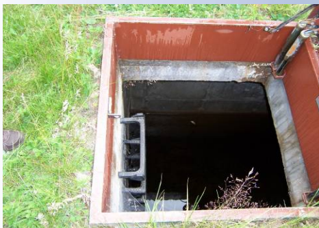
Hatch Entrance to the filter bed
