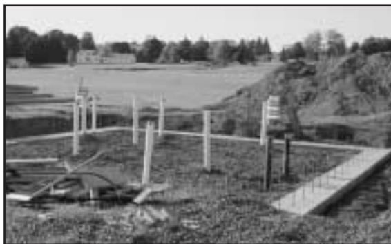
Foundation for the new plant in Westerlo
